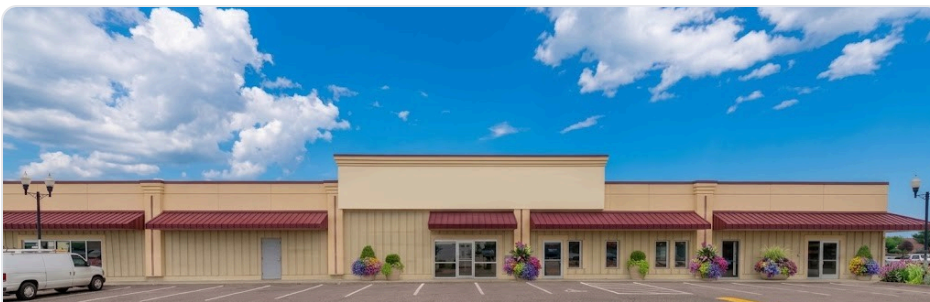
FRONTAGE AND PARKING FIELD
